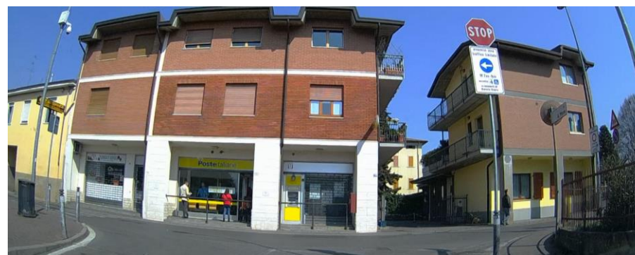
Figura 37 – ZTL – via San Rocco
